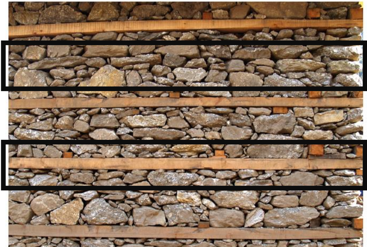
Figure 5-1 Stone layer (black box above) - Timber beam (black box below)
