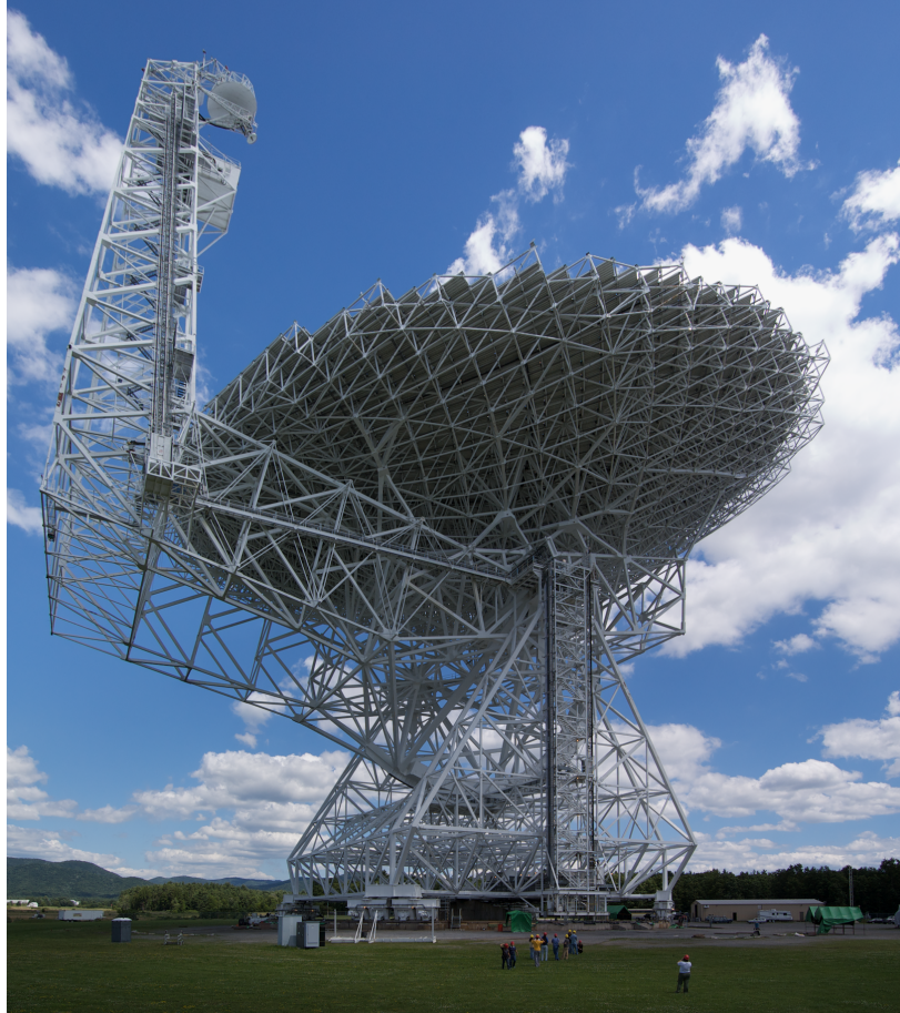
Figure 2.2: The GBT antenna, 148 m in height, has an arm supporting the primary focus that is cantilevered from behind the dish. In this way, the subreflector does not shade the primary mirror.
