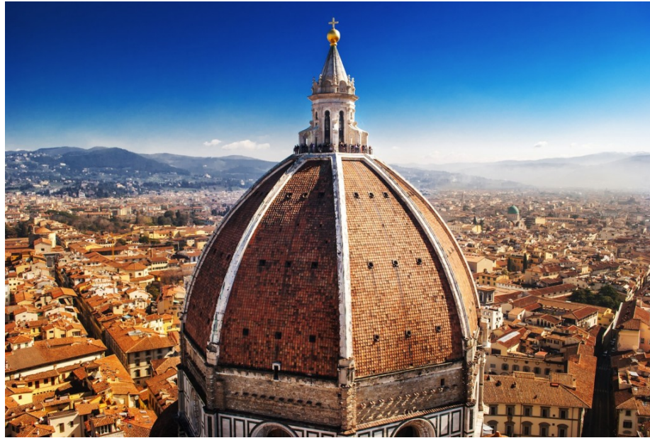
Figure 2.2. The Dome of Brunelleschi [2]
