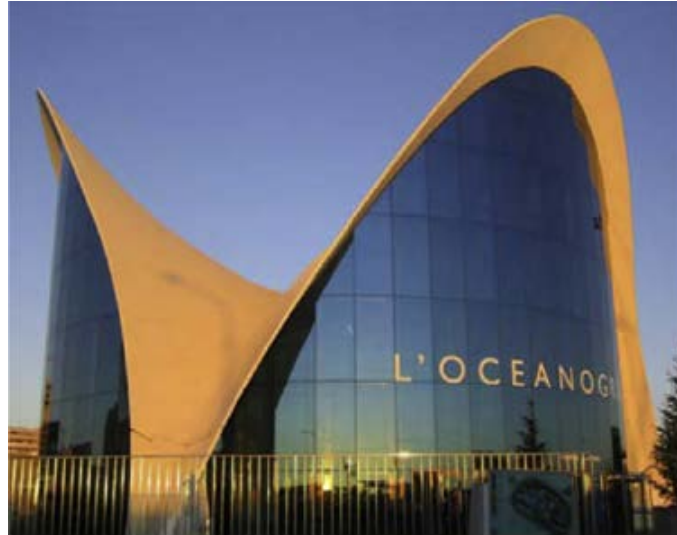
Figure 2.8. Hypar shell structure at the entrance of the Universal Oceanographic Park (Valencia, Spain) [23]
