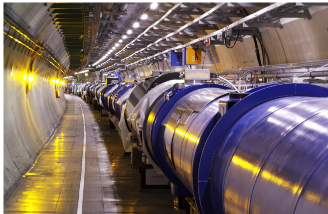
Figure 2.1: The LHC collider inside the underground tunnel (copyright CERN).
