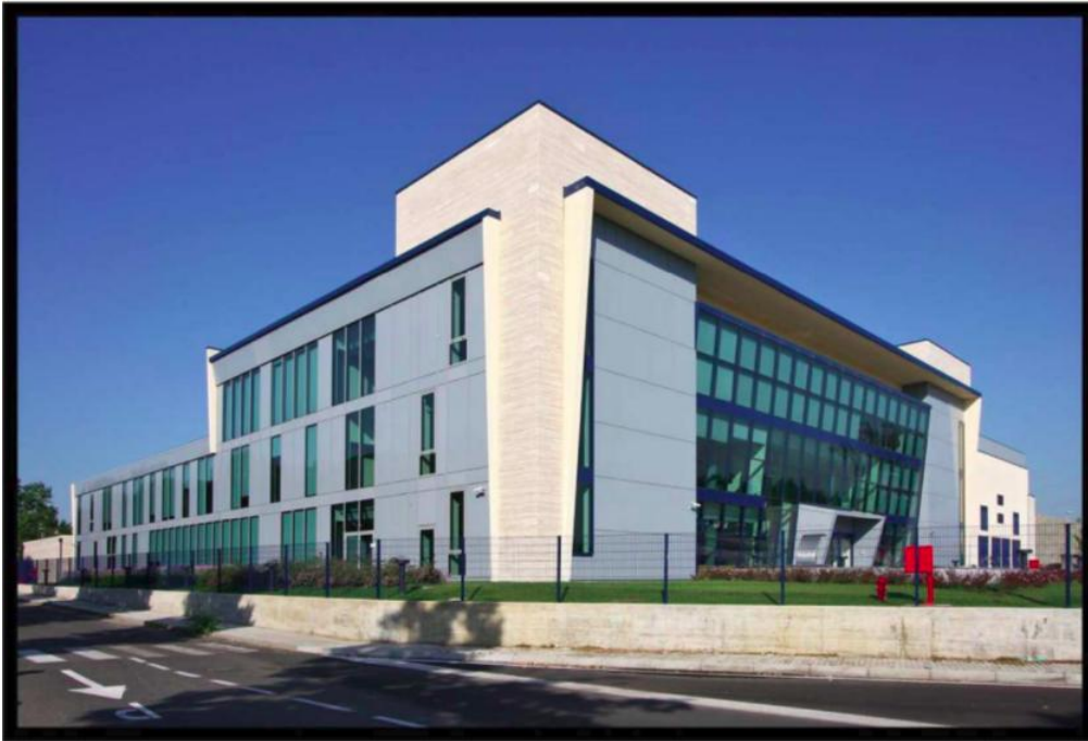
Figure 2.1: The CNAO hospital building in Pavia.
