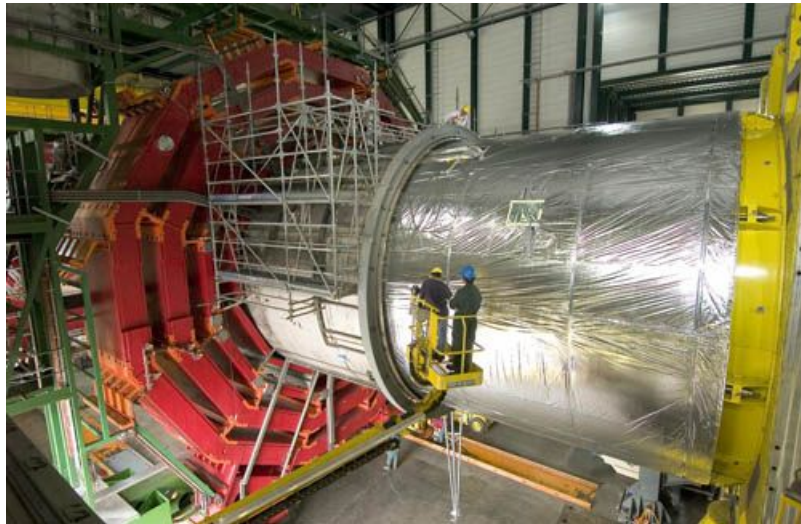
Figure 3.7: The CMS magnet during CMS construction.
