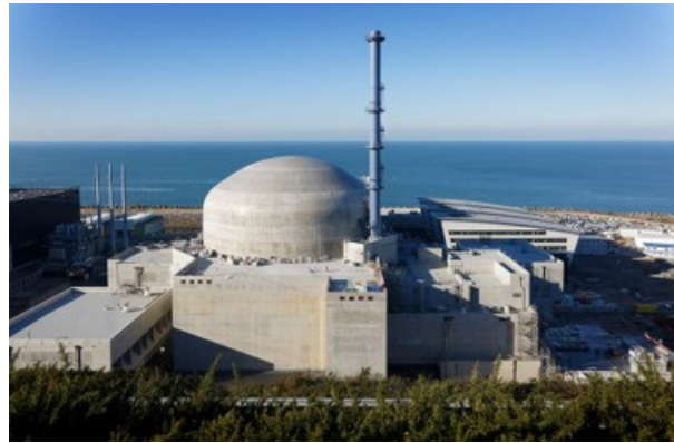
Figure 2.11: Overview of the Flamanville 3 EPR nuclear power plant unit upon completion of construction [7].
