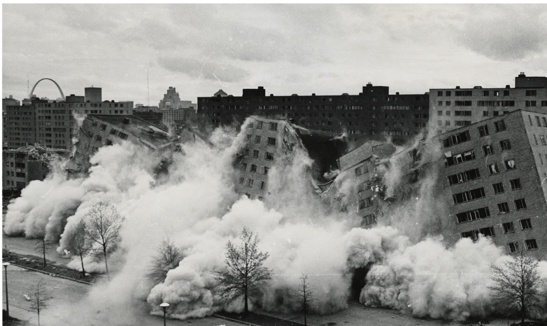
Figure 5: Demolition of Pruitt Igoe
