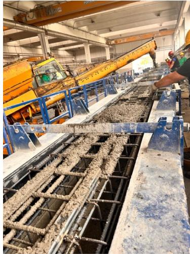
Figure 6. Casting process of precast pillar elements
