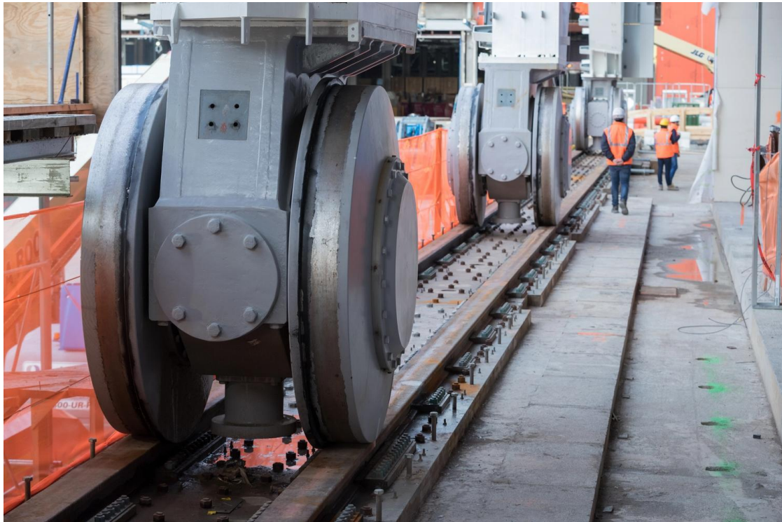
Fig 6.10: The Shed, Diller Scofidio + Renfro System of Rail and Rollers.(Archdaily, 2019)
