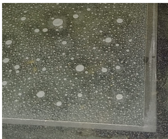
(b) TSP degradation after 1 month of submersion and recent drying.
