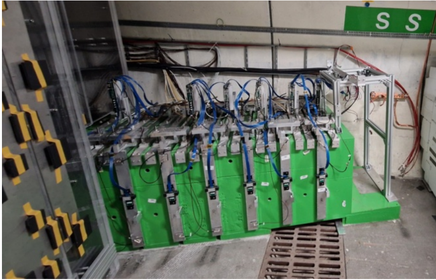
Figure 3.8: The mechanical support structure for MiniDTs and DS3-4, during the assembly.
