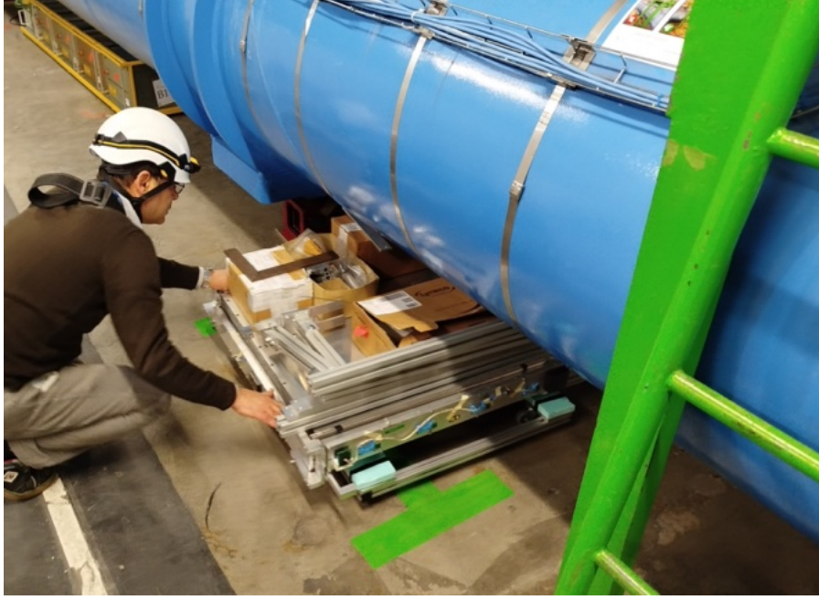
Figure 3.7: The material for the installation, including the MiniDTs and their (dis-assembled) mechanical support structure, were transported with trolleys low enough to cross the LHC beam pipe from below.
