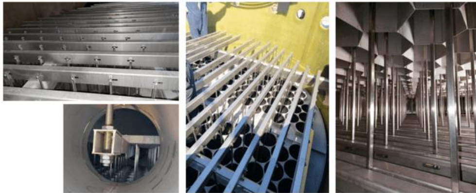
Figure 8: electrodes and support structure
