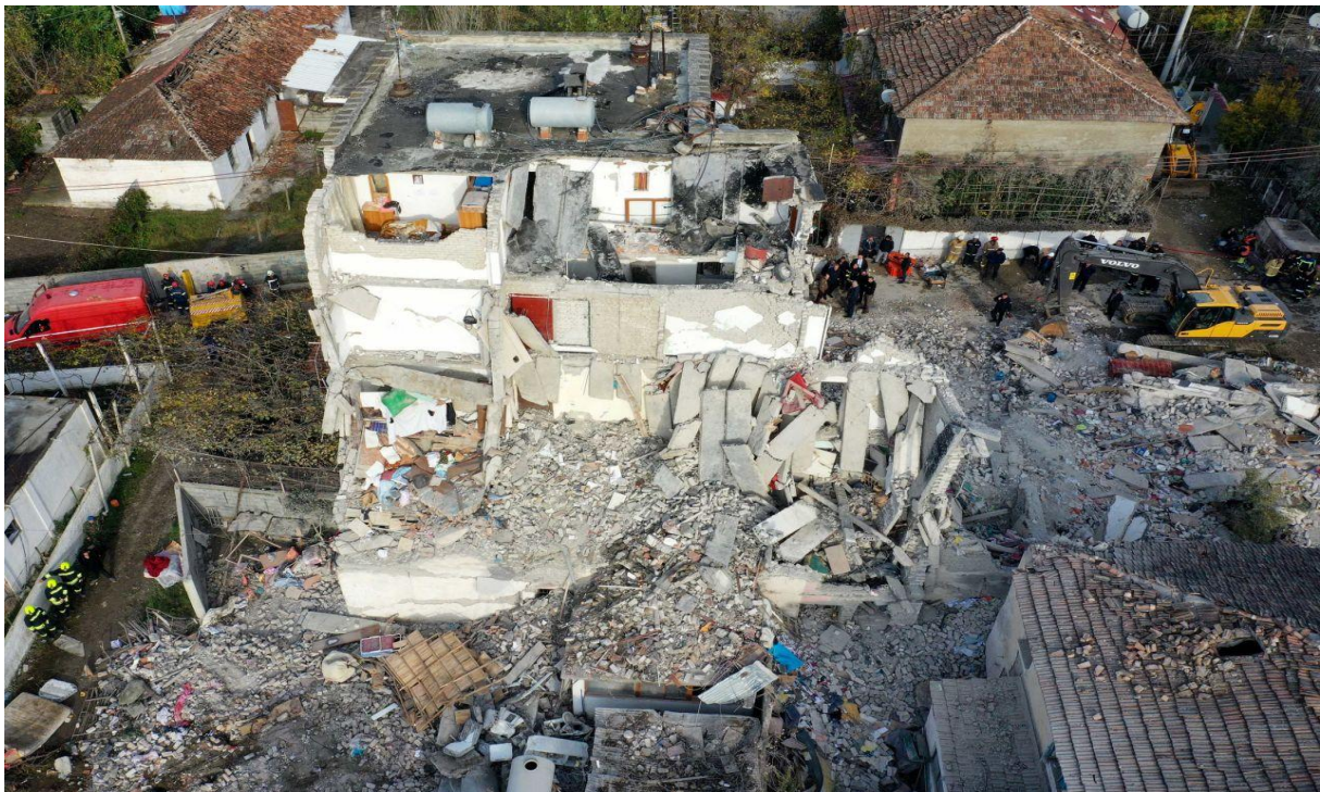
Figure 2.4. Picture captured after the Earthquake of the magnitude 6.4 near Durres, Albania (11.2019).
