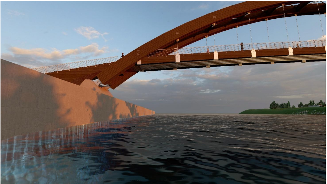
Rendering 7: Close-Up of the Arch Support on the Abutment Wall and Interface with the Concrete Base
