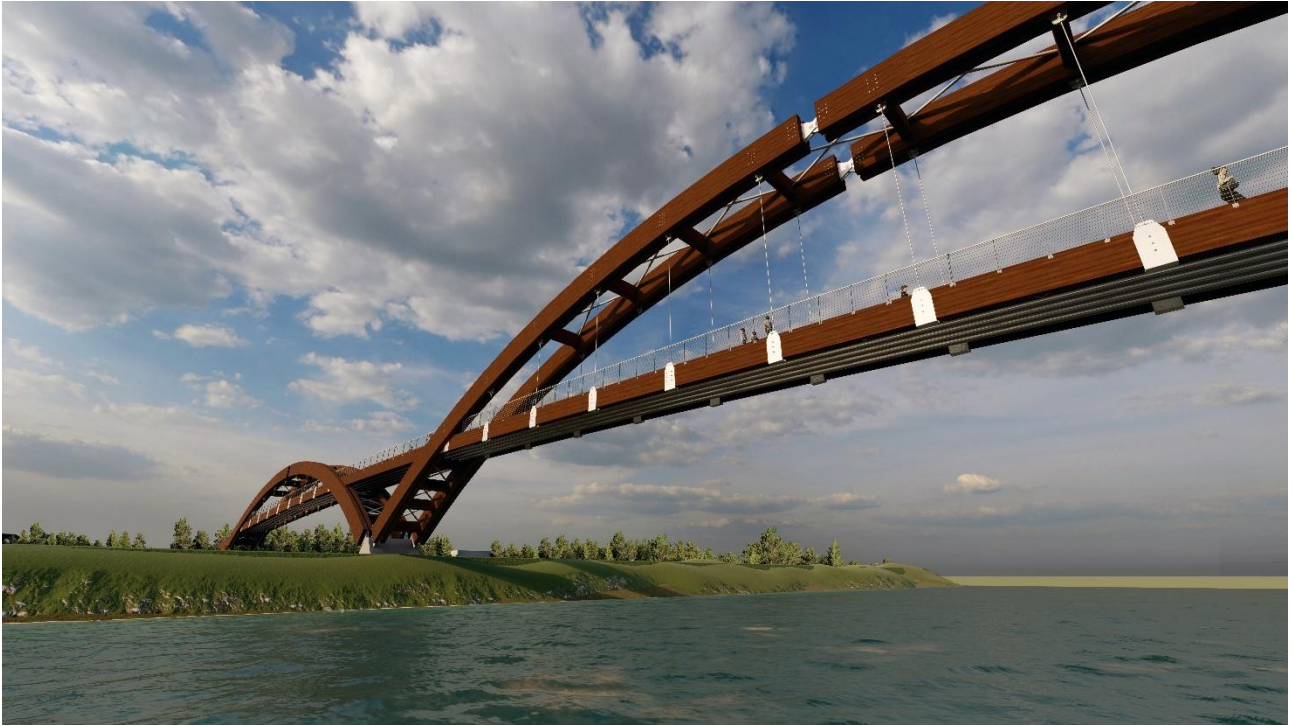
Rendering 5: Under-Deck View Emphasizing the Connection between Arches and Deck as well as the Arrangement of Hangers
