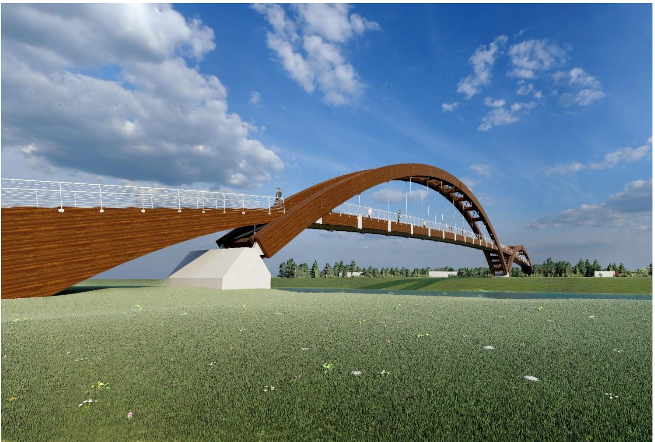
Rendering 6: Oblique View from the Riverbank, Illustrating the Articulation of the Support at the Foundation Level
