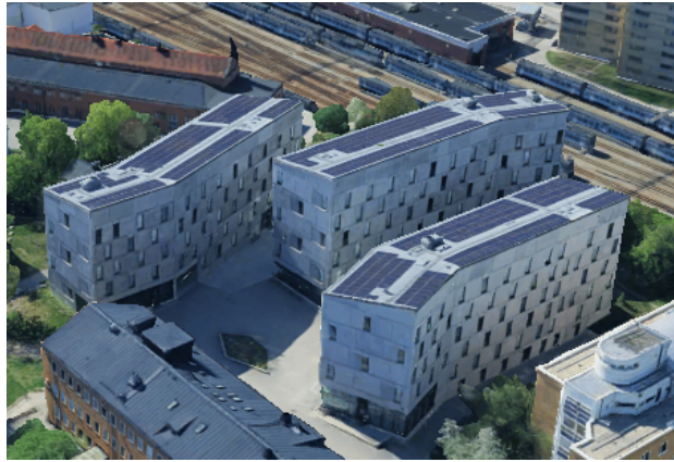
Figure 8: 3D view of the buildings heated by GSHPs connected to the borehole field [55]
