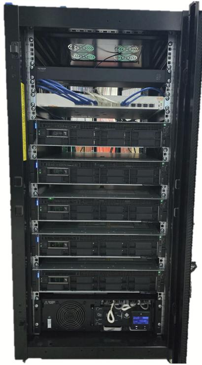
Figure 3: O-RAN Server Rack: Five Dell PowerEdge R750xs Units
