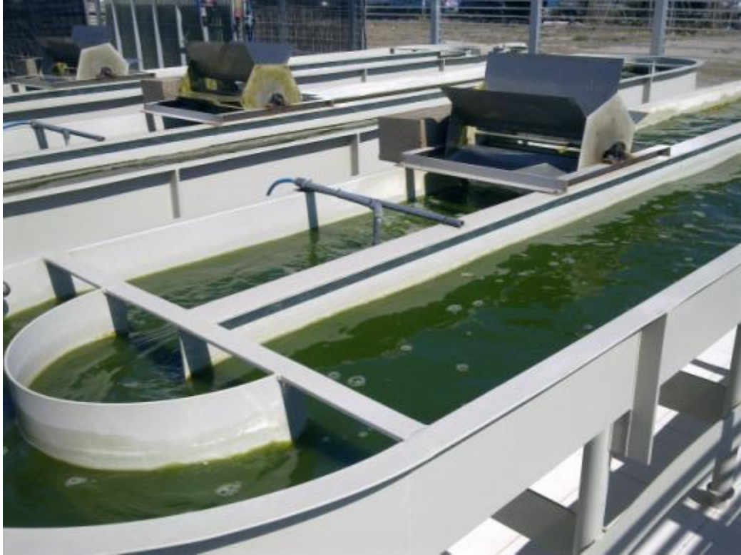
Fig. 1 – Pre-industrial open raceways in the campus pilot plant. (University of Almeria)
