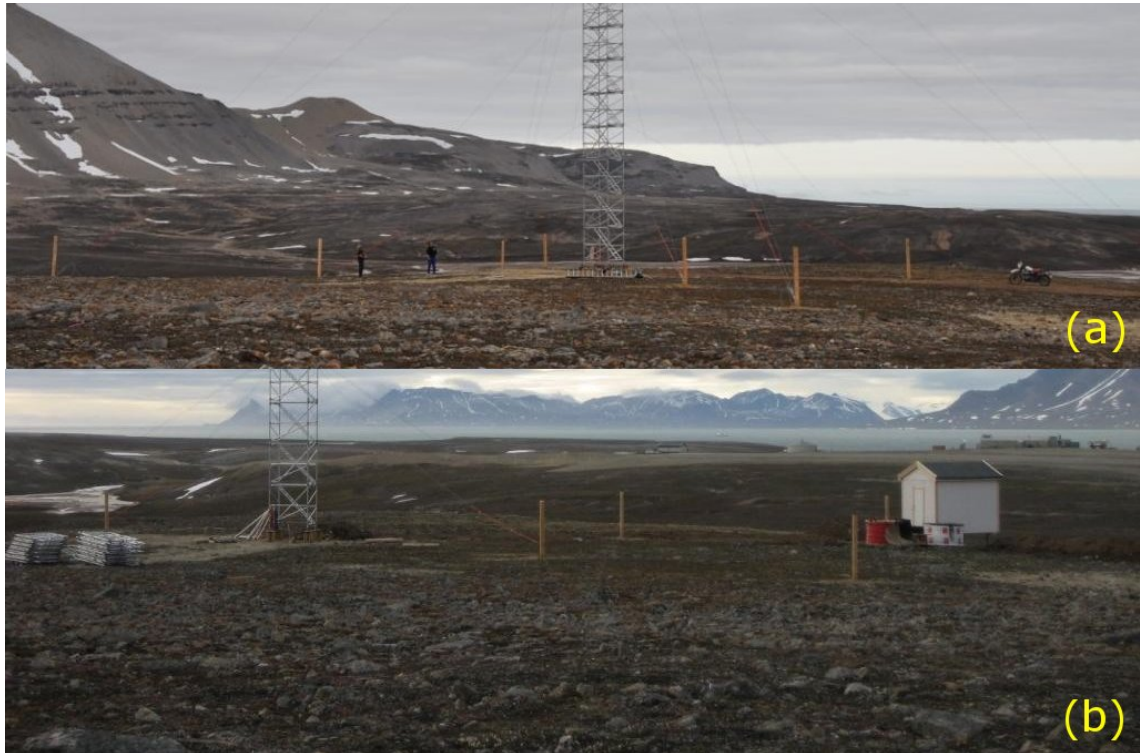
Figure 2.3: The CCT site as viewed from south-east (a) and from south (b) during the erection of the tower structure (ISAC-CNR, 2014).
