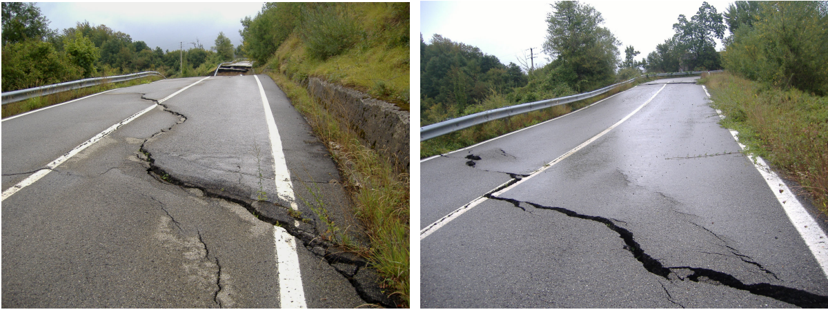
Figura 117 - Tension crack in sinistra nicchia, Tension crack in destra nicchia.
