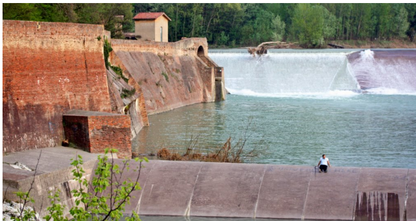
Fig. 5.8 – The river Reno run throughout the city: here at a medieval lock (ph. Carlo Pelagalli).
