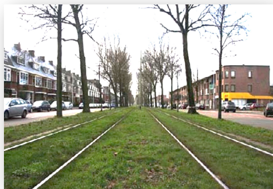
Fig. 3.3 – Green tramway tracks at Le Hague, The Netherlands (Ruijs, 2012).
