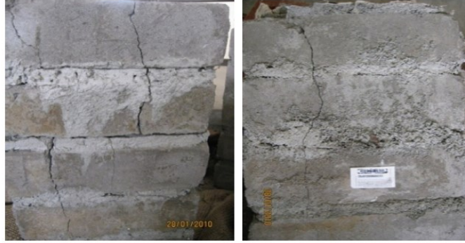
Figure 4.57: Failure of masonry brick prism under an axial loading (Christy, 2013).
