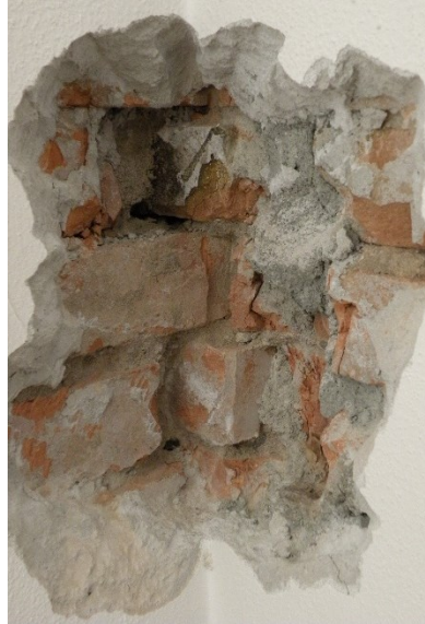
Figure 7.3: Visual inspection of the walls connection.
