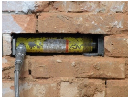
Figure 4.18: Hydraulic Jack placed instead of the removed masonry unit.
