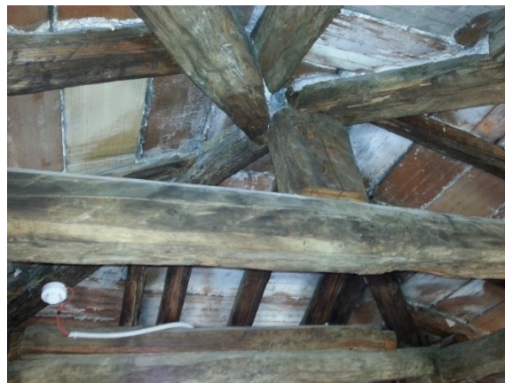
Figure 7.21: Timber truss supporting the sloped roof.
