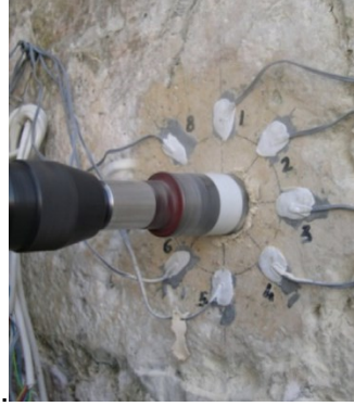
Figure 4.52: The application of Hole-drilling test (Lombillo et al., 2013).
