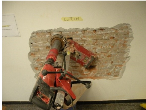
Figure 4.26: The application of core drilling equipment.
