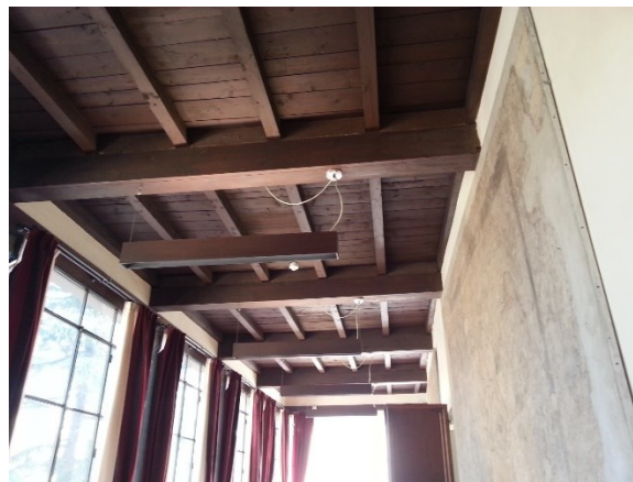
Figure 7.22: Timber beams supported by the walls.
