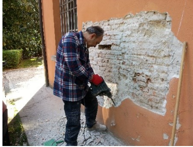
Figure 4.17: Removing plaster by electrical hammer as preparing phase of shear test.
