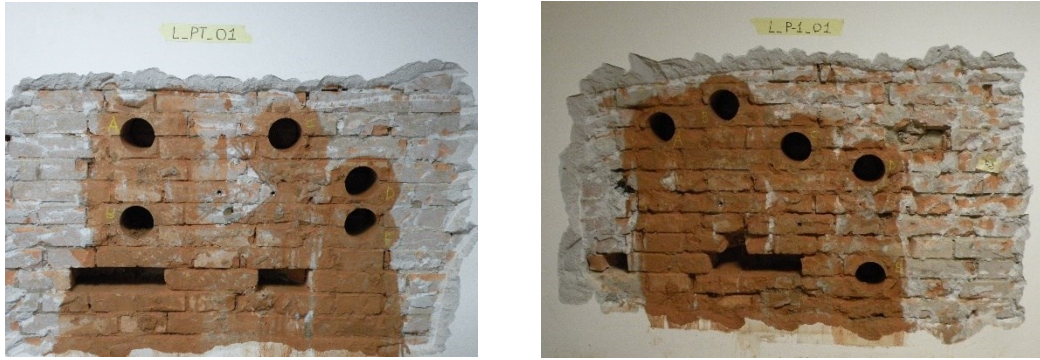
Figure 7.1: The masonry walls, where the specimens have been executed (L_PT_01), (L_P-1_01).
