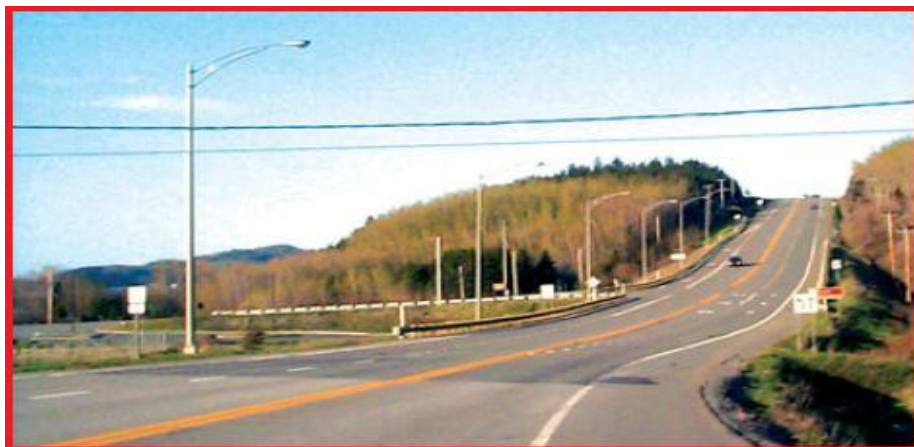
Figure 6.29: Combination of intersection and climbing lane at uphill grade to be avoided in the design
