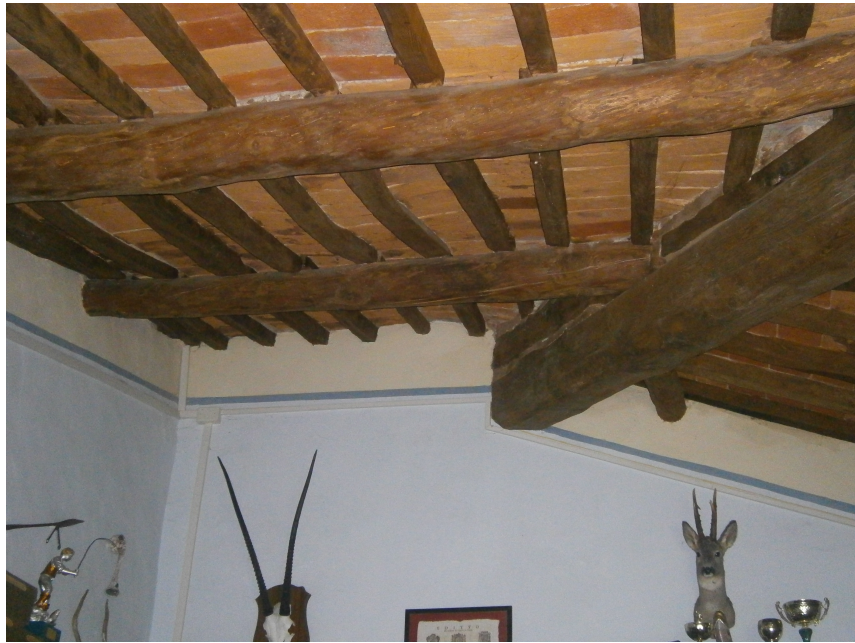
Picture 13. Detail of an Inner connection of first floor roof
