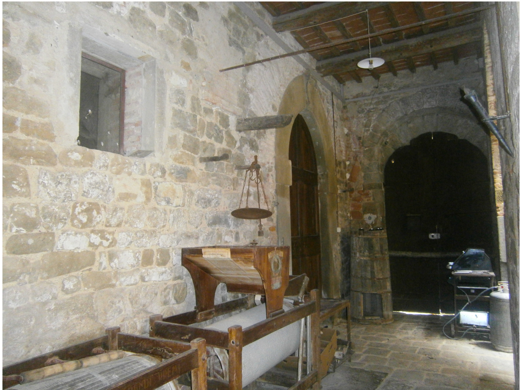
Picture 25. Example of ordinary masonry
