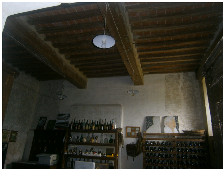
Picture 5. Two orders timber beam slab 1
