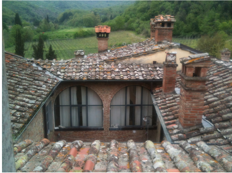
Picture 10. First floor roof connections
