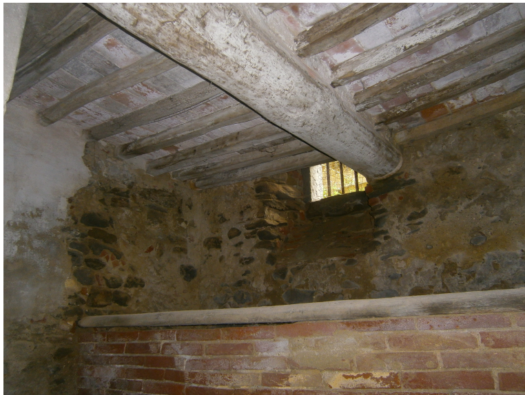
Picture 7. Two orders timber beam slab 3
