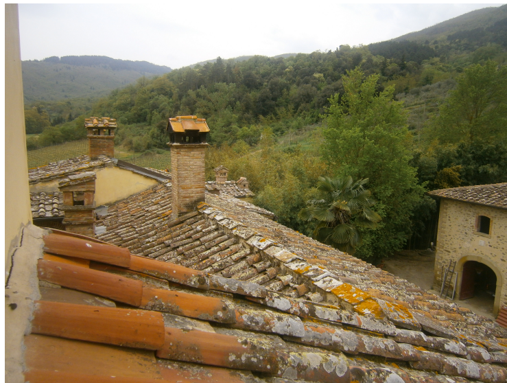
Picture 11. Second floor roof connections
