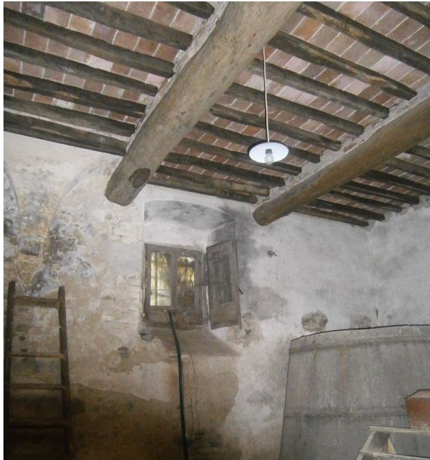
Picture 6. Two orders timber beam slab 2
