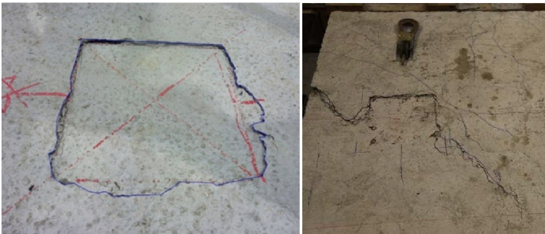
Sinking of the loading plate inside the concrete on the compressed side
