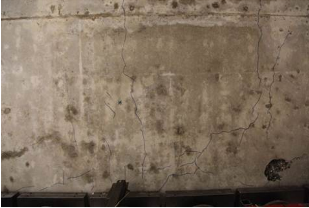
Cracking pattern at the bottom face for S25T1 slab
