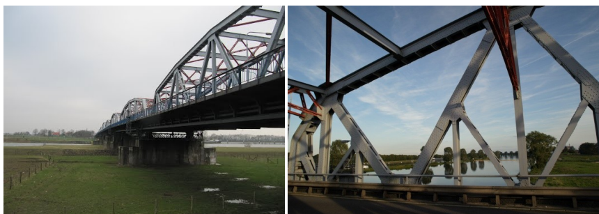
The John S. Thompson-Brug is a bridge over the Maas River, in the province of North Brabant in the Netherlands. The bridge was built in 1929 as part of the main road between 's-Hertogenbosch and Nijmegen. It still carries that road, now signed provincial route N324.
