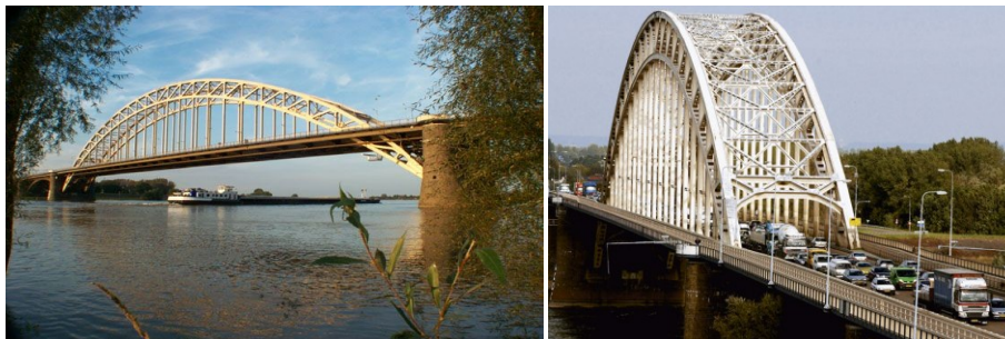
The Waalbrug is an arch bridge, with a full length of 604 m, over the Waal River in Nijmegen, Netherlands. The bridge was opened in 1936 and in the last years it is affected by large traffic jams during the rush hours. Because of its crucial aspect in regional traffic it has been difficult to renovate the bridge.
