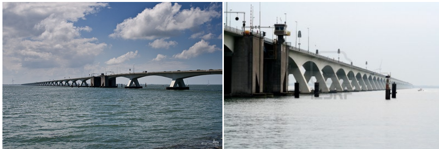
The Zeeland Bridge (Zeelandbrug) is the longest bridge in the Netherlands. With a structure made mainly of reinforced concrete and a total length of 5022 m, it connects the islands of Schouwen-Duiveland and Noord-Beveland in the province of Zeeland. The Zeeland Bridge was built between 1963 and 1965.
