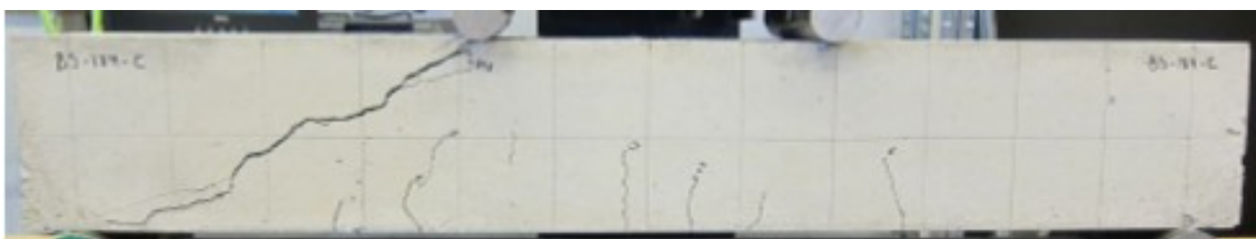
Shear crack in reinforced concrete beam at failure
