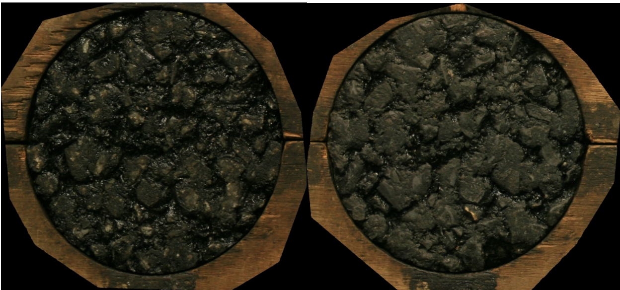
Figure 6.4 – Reconstruction of texture pre and after trafficking using Topcon Image Master
