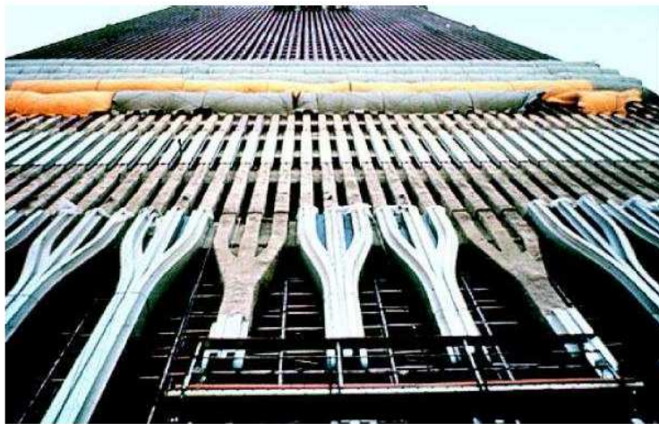
Figure 14. Base of exterior wall frame. FEMA report 2002. FEMA report 2000
