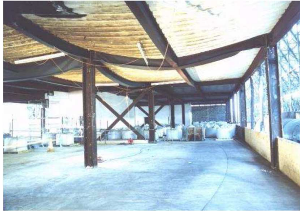
Figure 23. Test fire at Cardington FEMA report 2000
