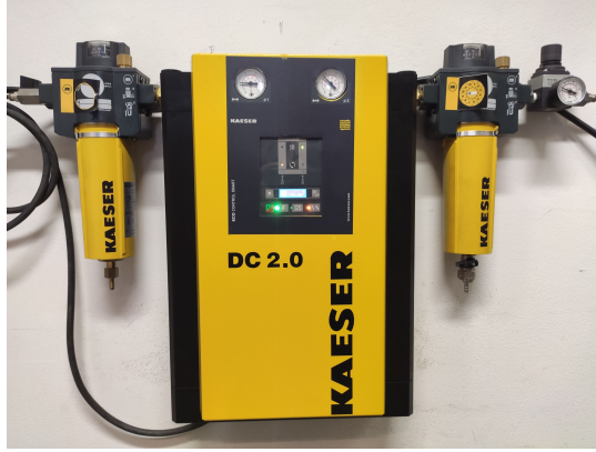
Figure 3.3: The KAESER DC 2.0 heatless regenerative desiccant dryer.
