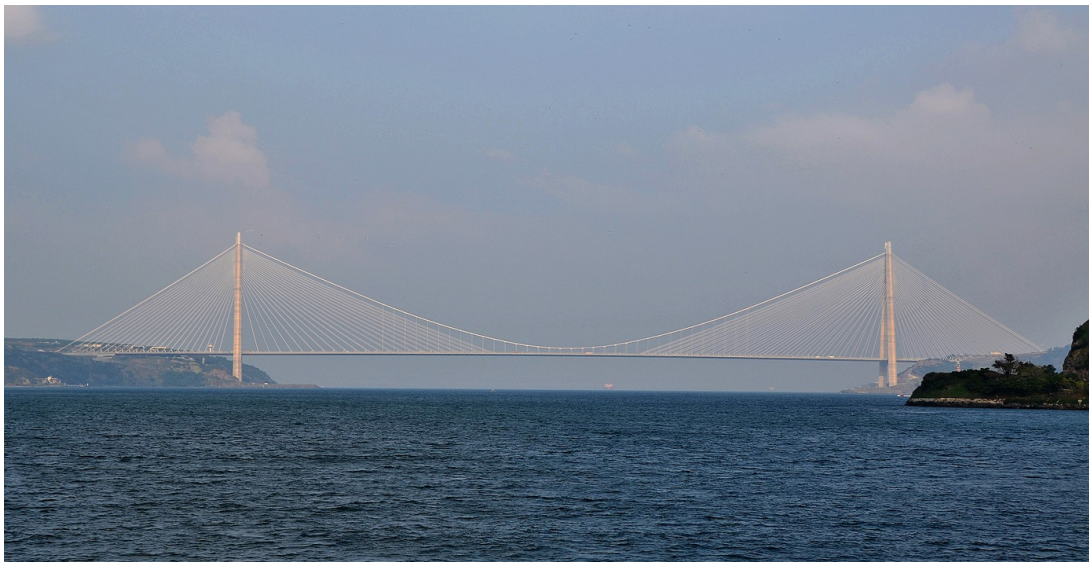
Figure 32: View from the south of the Third Bridge over the Bosphorus
