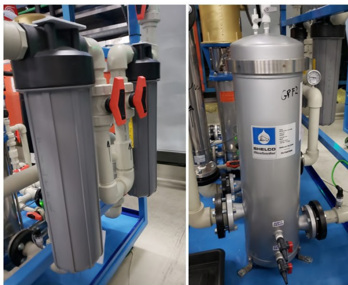
Figure 4.7: Particle filters of the GdWPS. On the left, two filters placed in parallel (GPF4 and GPF5); on the right, GPF2 (of different type).
