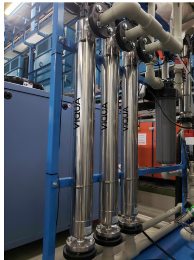
Figure 4.10: Three UV lamp units disposed in parallel to form GTOC2. They are placed before the ORT resin.
