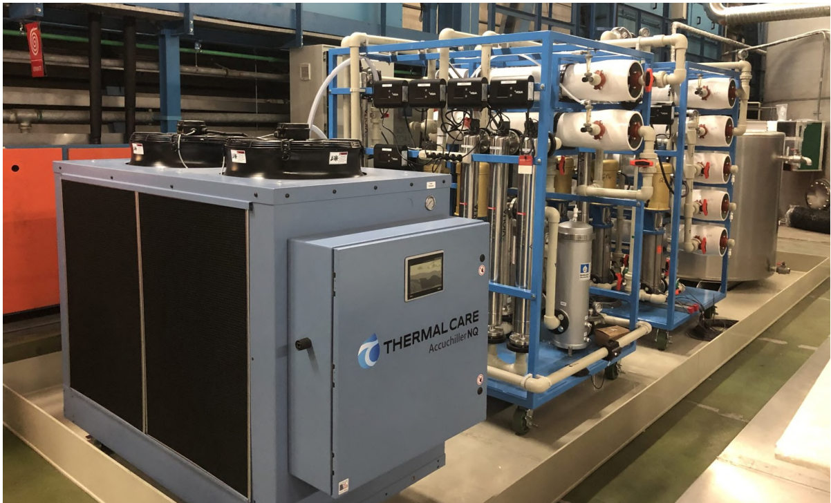
Figure 4.1: Picture of the Gadolinium-water purification system, placed close to the XENON tank.
