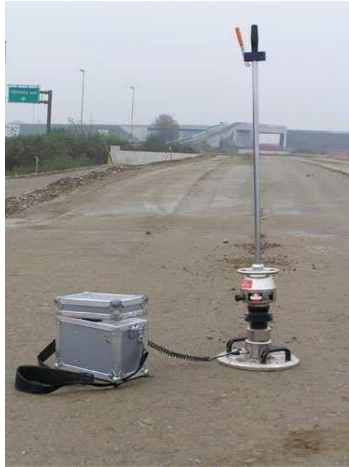
Fig. 4.32 – Light Falling Weight Deflectometer .
