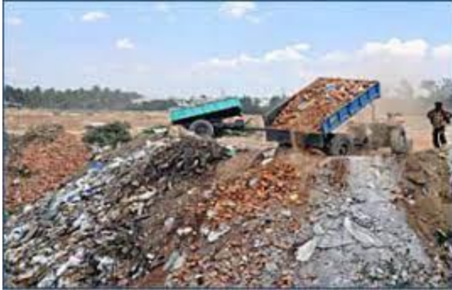
Fig 8: Disposal of C&D waste into open area
