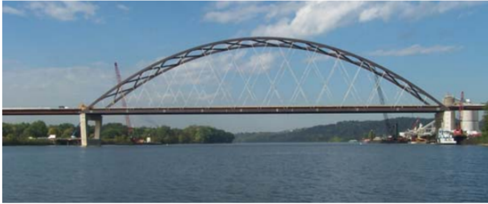
Blennerhassett Island Network Tied Arch
