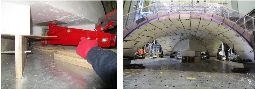
Figure 33: Formwork removal.
