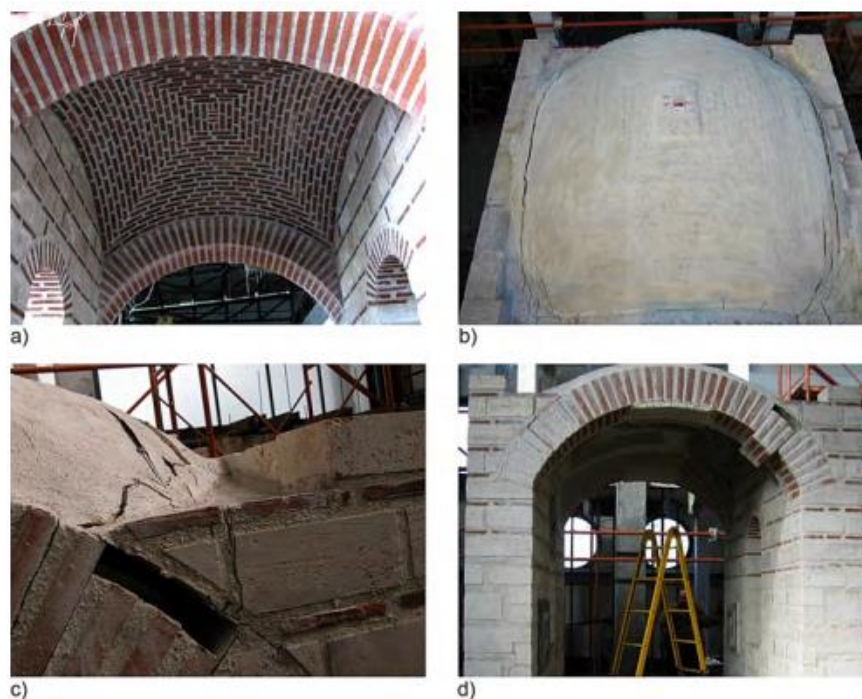
Figure 20: Tested cross vault in NTUA: a) interior view; b), (c), (d) damages at the end of the test.
