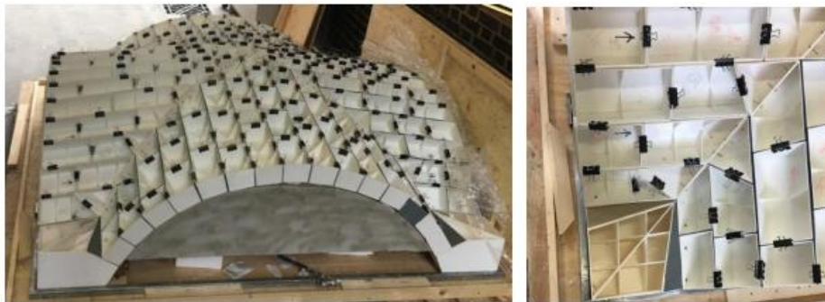
Figure 31: Pre-assembly of the vault with empty blocks.
