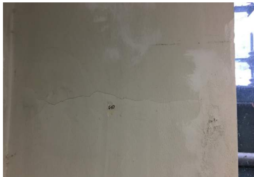
Figura 13: Fessura media F10.
