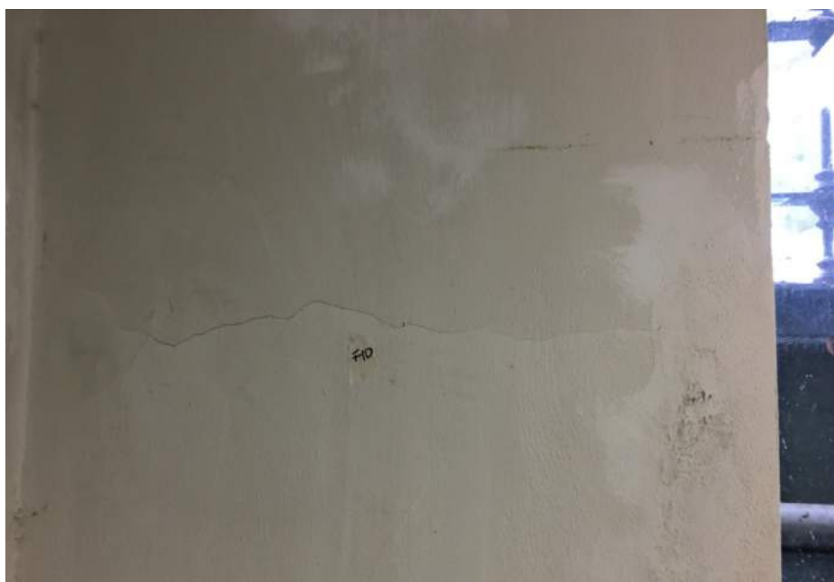
Figura 5.12: Fessura media F10.
