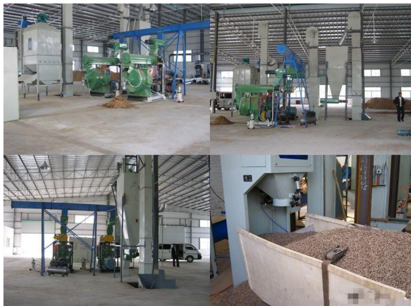
Figure 11 A pellet plant in Portugal (available at http://www.biomasspelletplant.com/news/pellet-market-portugal.html )
