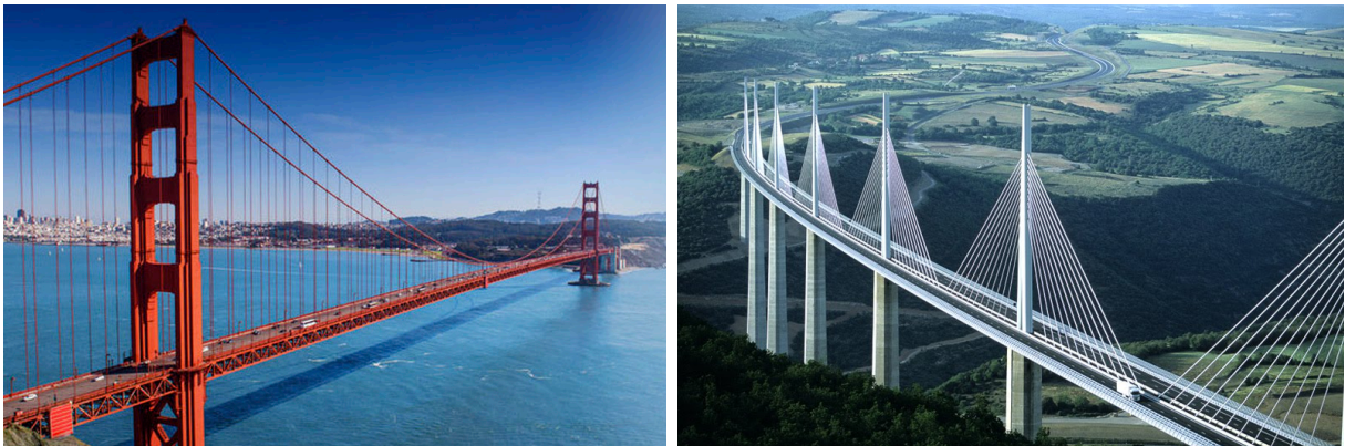
Figure 1.1: Golden Gate Bridge (San Francisco, US) and Millau Viaduct (Creissels, France).
