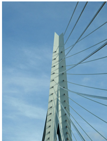
Figure 1.2: Particular view of a cable-stayed bridge showing the sag of stay cables.
