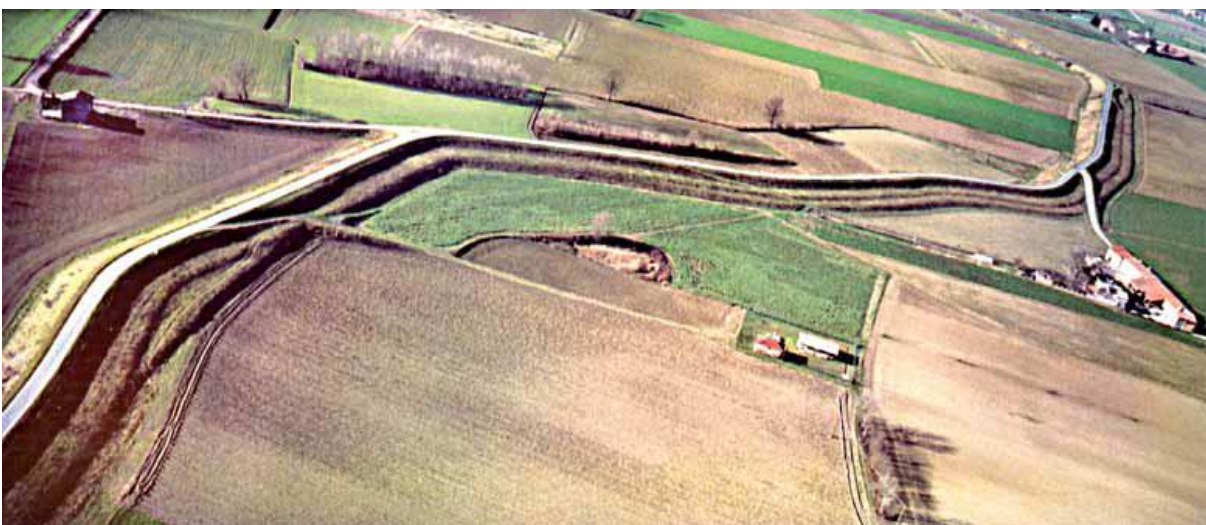
Figure 189: View of the main levee system in Cremona Province (V. Ferrari, F. Leandri, and C. Milesi, 2008)
