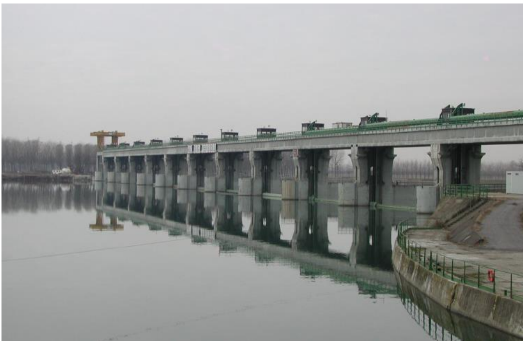
Figure 16: The Isola Serrafini dam (AdbPO, 2005)
