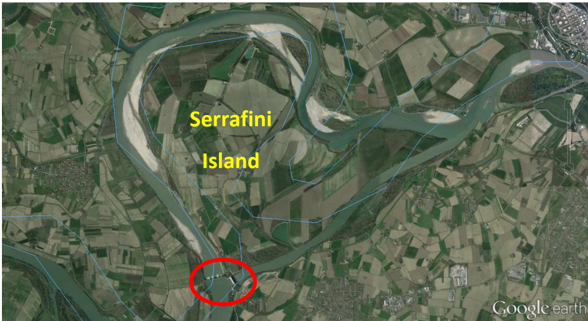
Figure 15: Localization of the dam of Isola Serrafini (Google earth)
